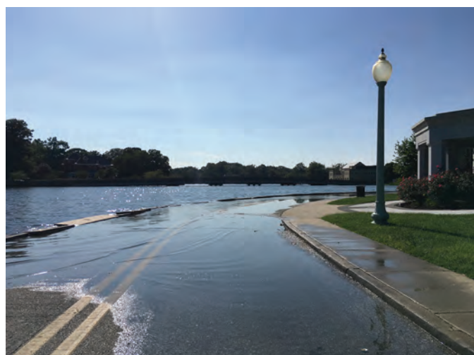
FIGURE 2. United States Naval Academy sunny day flooding: Ramsey Road on September 20, 2017, during high tide. The road frequently floods and has to be closed by security. This impacts memorial ceremonies and internments at the Columbarium, as well as impeding traffic to and from the faculty parking lots on Hospital Point. Historic Hubbard Hall is in the background. Photo courtesy Dr. Angela Schedel, USNA alumnus.
