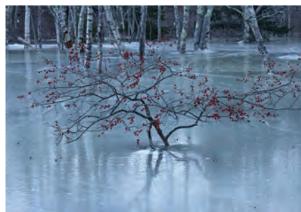
FIGURE 4. Images from a winter flood of Great Meadow following a large rain-on-snow event that froze while at flood stage. This type of flooding has become more common in recent years, caused in part by an undersized culvert at the outlet to Great Meadow. Photos courtesy of Jeff DiBella (top) and Julia Walker Thomas (bottom).
