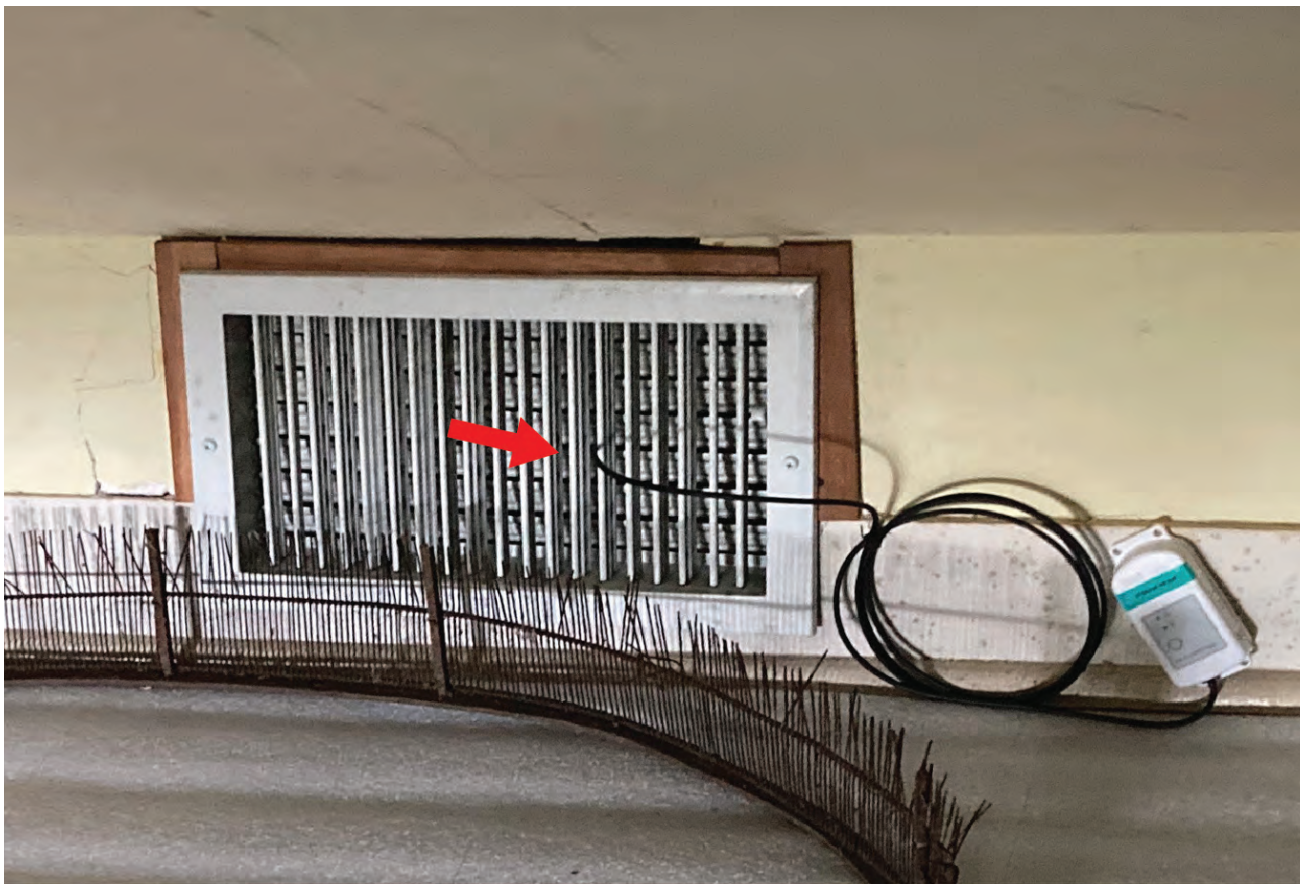
FIGURE 3 (above). Monitoring differential pressure between interior and exterior. FIGURE 4 (below). Monitoring temperature and relative humidity at supply register. DAVID BITTERMANN
