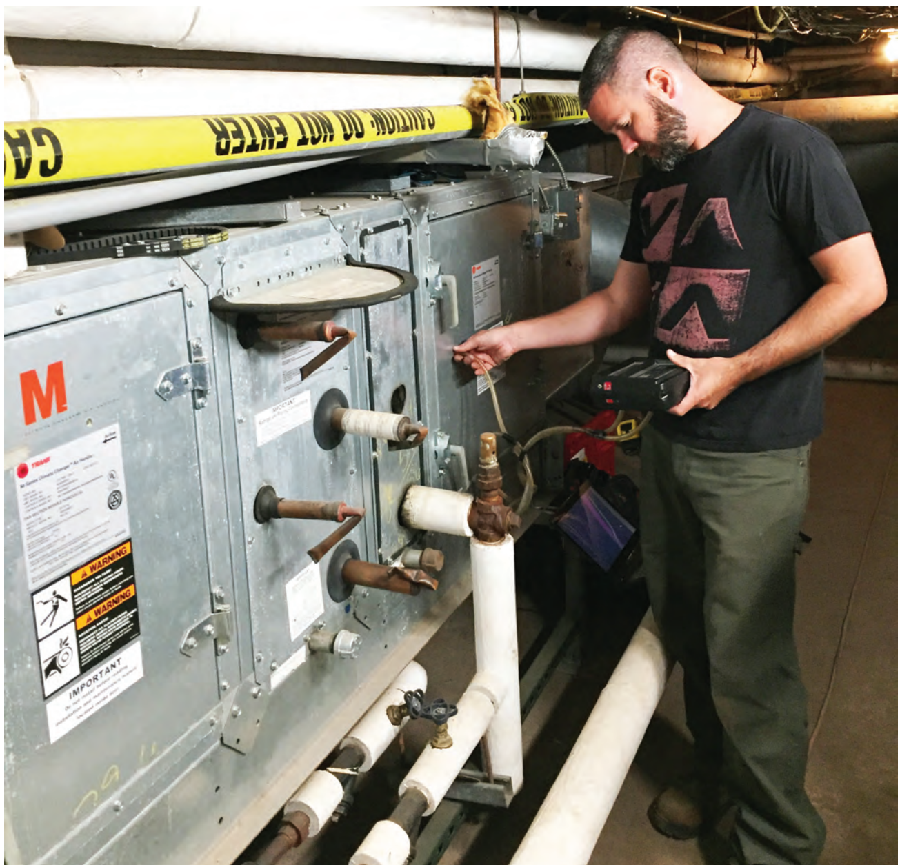
FIGURE 10 (above). Thermal imaging at Sagamore Hill. STEVEN WEINTRAUB, ART PRESERVATION SERVICES FIGURE 11 (below). Measuring static pressure and airflow at air handler. DAVID BITTERMANN
