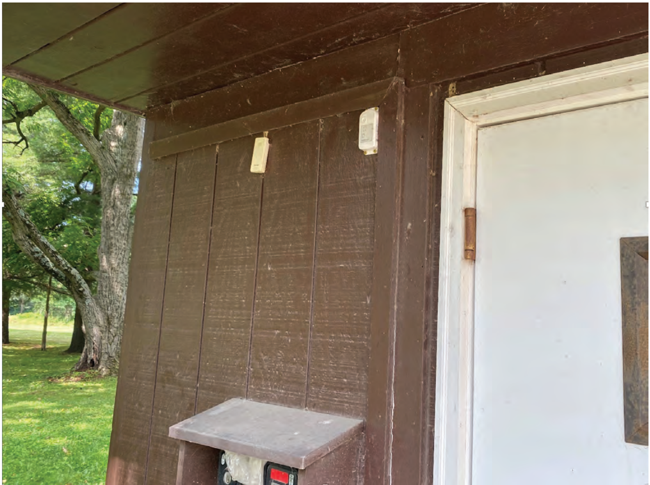
External temperature gauge mounted on maintenance facility immediately behind Lindenwald. NATIONAL PARK SERVICE
