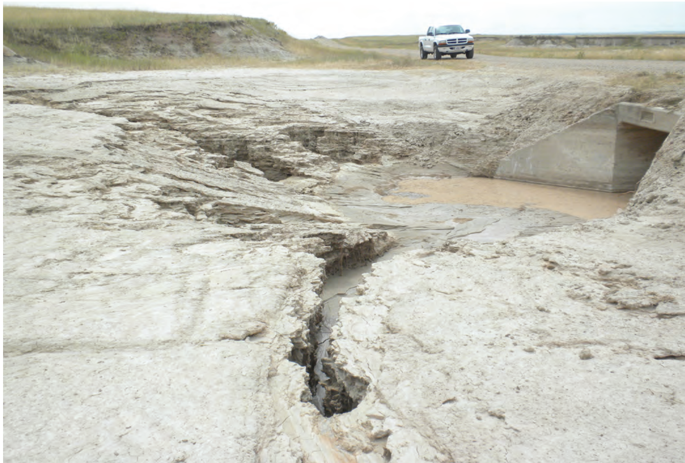
FIGURE 1. ABOVE A box culvert and associated drainage along Old Interior Road that was cleaned and shaped by the Maintenance Division in 2011. A system of box channels was created by subsequent precipitation. BELOW The same drainage system in 2023. The box channels are still present but erosion at the inlet of the culvert has abated, allowing vegetation to proliferate.
