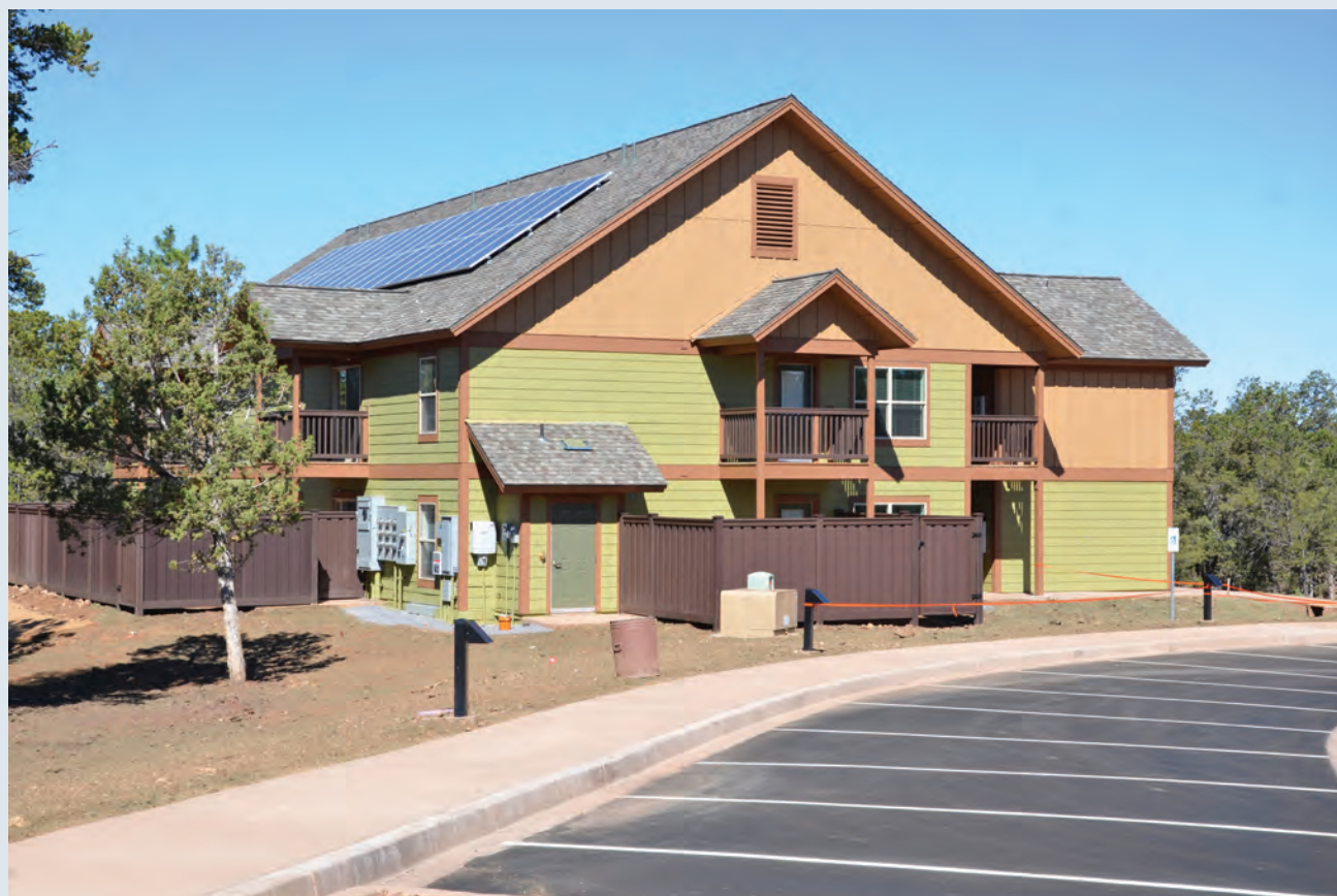
Multi-family employee housing at Grand Canyon National Park. NATIONAL PARK SERVICE
